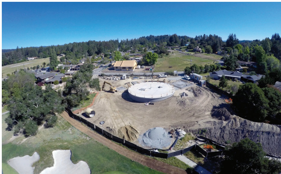
Water works: A bird’s-eye view of Pasatiempo Golf Club’s new water storage tank, water treatment facility and pump station in May. The system, which recycles treated wastewater from the nearby city of Scotts Valley, Calif., came online in September. Photo courtesy of Justin Mandon
